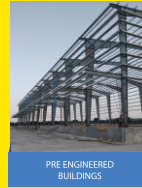
PRE ENGINEERED BUILDINGS
