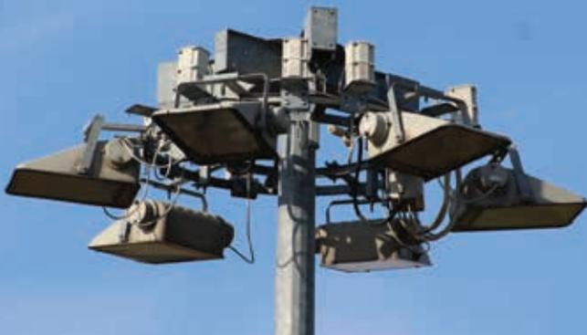
Lowering headframe masts allow the headframe to be lowered with a winch and are ideal for accessing headframes at ground-level when space around the mast is tight. These lowering headframe masts provide easy maintenance access at mast base and offer additional features such as optional headframe latching. Benefits include reducing risks of multiple internal cable-snagging problems by using a single multi-core electrical cable system for up to 12 floodlights.
