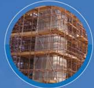
SCAFFOLDING & FORMWORK SYSTEM
